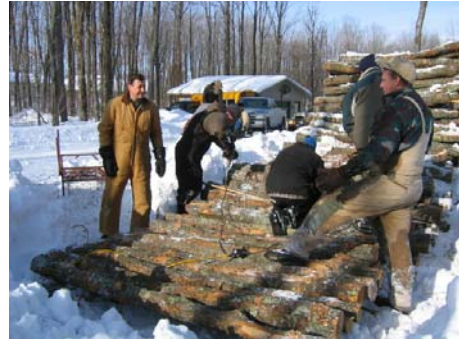
FOG members, DNR employees, and other volunteers work together to prepare the timber frames that will become fish cribs.
