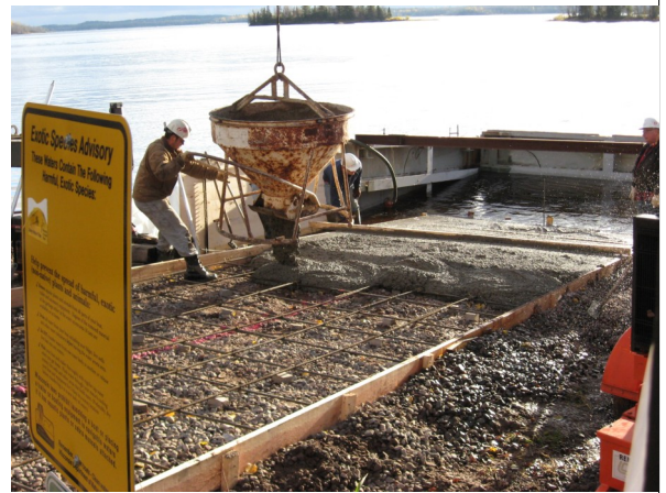
Xcel work crew pouring the boat landing's concrete base.
